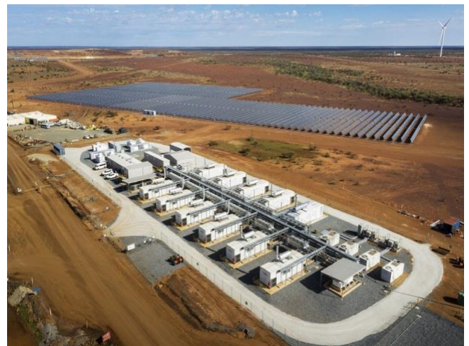
The 4 MW of solar panels and associated storage at Agnew Gold Mine 7
